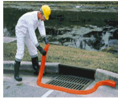
**Storm Drain Covers/Mats** – These devices are placed on top of the storm drain cover grate, creating a quick seal, thus preventing wastewater from entering the storm drain system. Storm drain covers/mats (magnetic vinyl mats, PVC drain covers, polyurethane mats, and others) allow wastewater to accumulate on top of it until the pressure washing activity is complete
